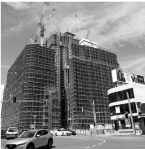
JQZ under construction construction
