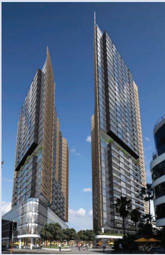
St Leonards Sq 472-486 Pacific Highway, St Leonards Lane Cove LGA Under Construction 539 apartments
