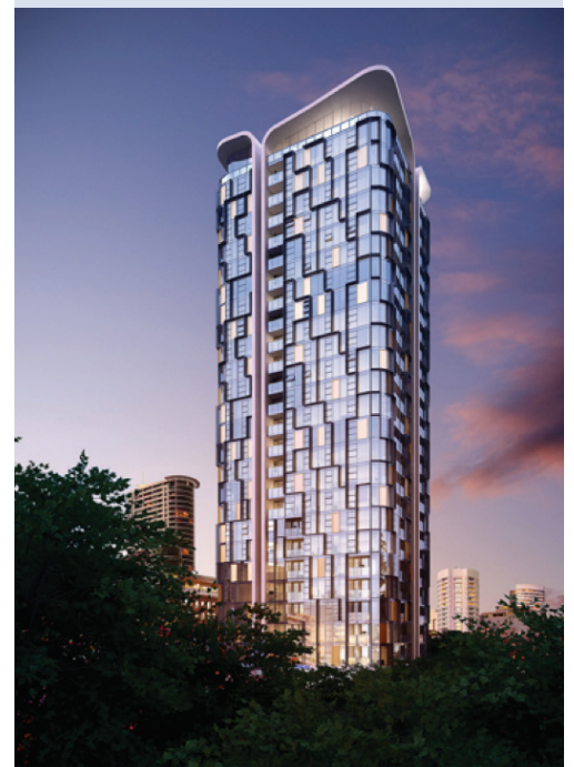
Embassy Tower 1 Marshall Ave, St Leonards Lane Cove LGA Under construction - 269 apartments
